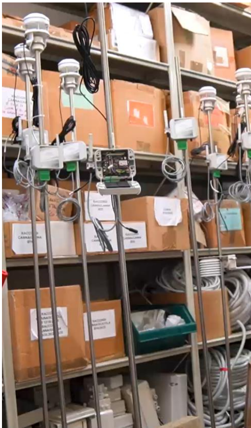
EE071, METER ATMOS22, Grillo BEE (MOUNTED SYSTEM)
